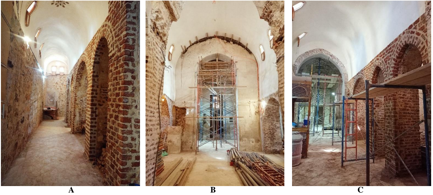
Figure 12. A, B, C represents the removal of damaged layers of mortar from the walls and columns at the church nave (Photo: Father Matta Anba Bishoy)
