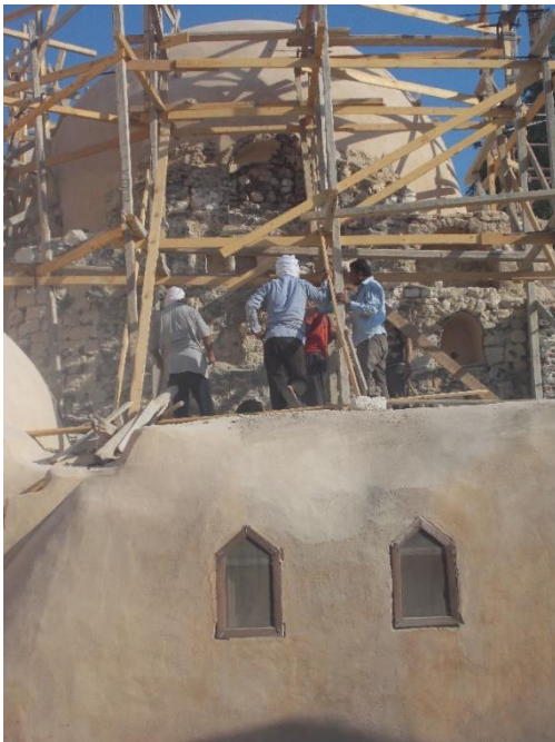
Figure 9. Removing the damaged mortar layer due to rain and floods
