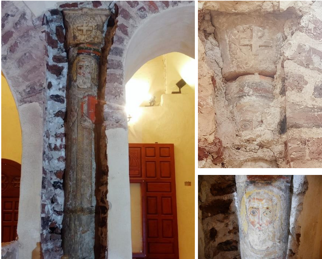
Figure 16. One of the marble columns discovered in the nave of the church, in good condition (photo: Father Matta Anba Bishoy- Emil Henin)
